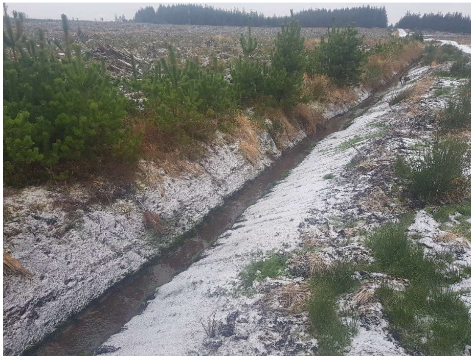
FIGURE 4-22: SUB-COMPARTMENT 33196S-2 ADJOINING FOREST ROAD DRAIN
