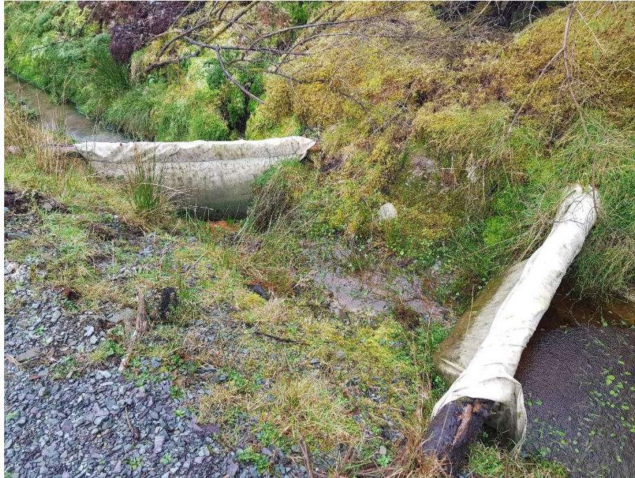
FIGURE 4-23: SUB-COMPARTMENT 33196S-2 ADJOINING FOREST ROAD DRAIN SEDIMENT TRAPS USING LOGS AND GEO-TEXTILE
